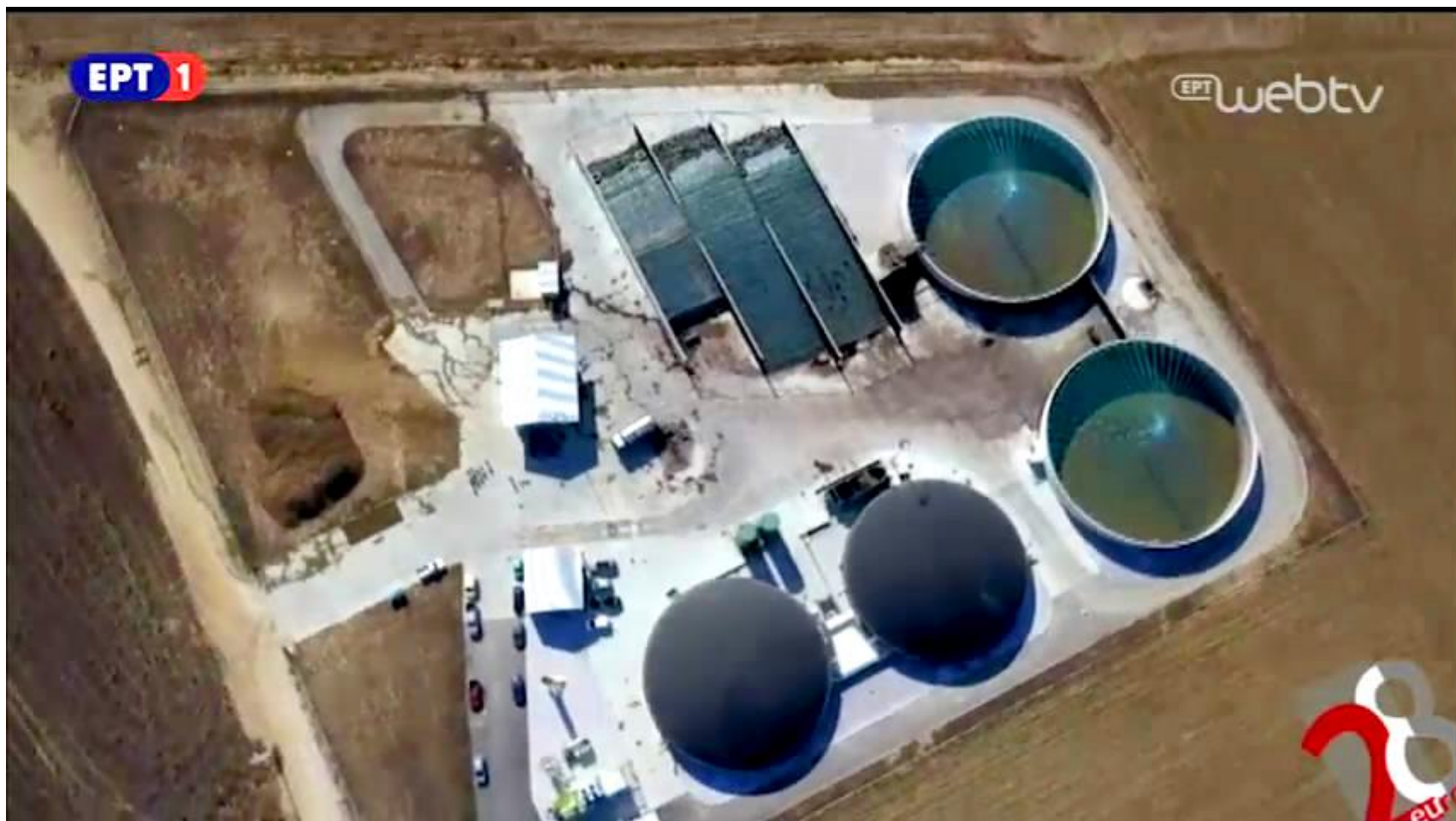
Panoramic photo of Biogas Lagada
