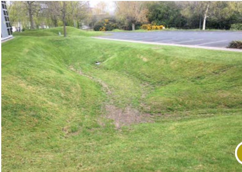
Figure 14: Detention Basin - City West, Dublin
