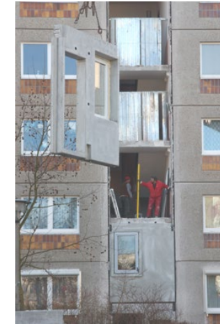
Installation of elevators
