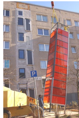
Installation of elevators
