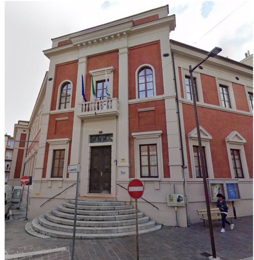
'Maria Montessori' University Student House after renovations
