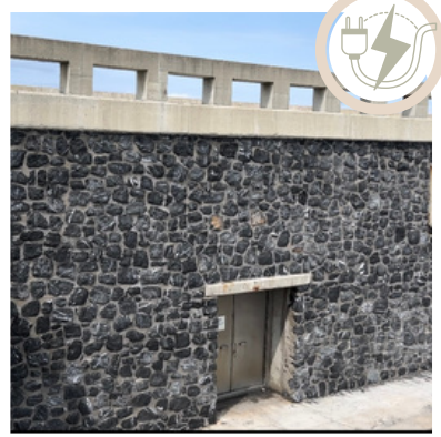
ENTRANCE TURBINE ROOM
