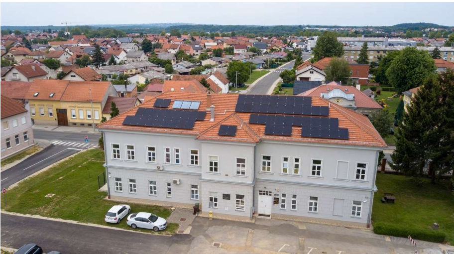
Solar power plant - 3 administrative buildings -20kW
