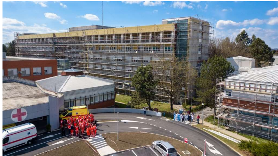
Energy efficient renovation - Eprim decrease of 56,43%, CO2 56,98%
