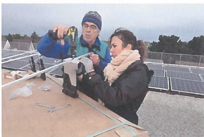
Participatory work site - installation of photovoltaic panels
