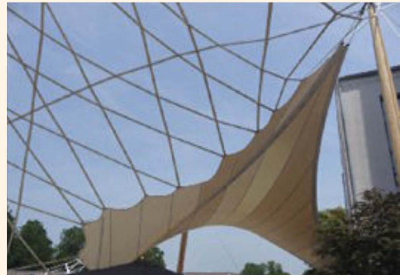
Textile-based membrane structure
