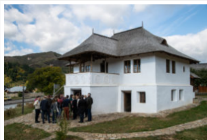
Study visit at The House with the Coat of Arms in Chiojdu, Romania. Photo_ Vlad Băscă
