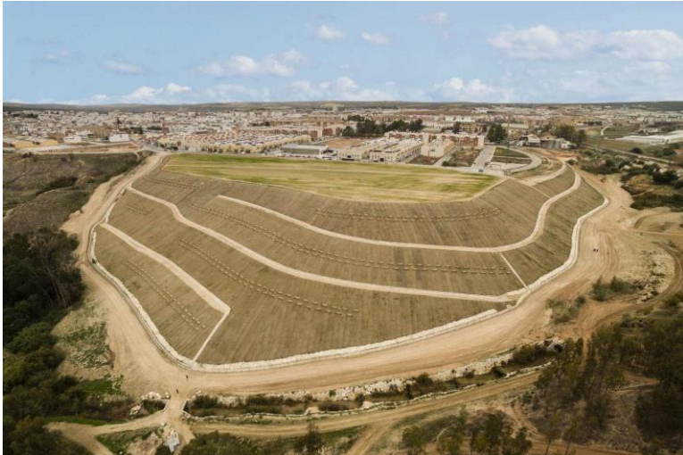
Image: closed and remediated landfill Puente Genil in Andalusia (from [08])
