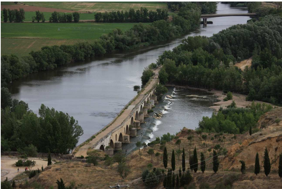
Main bridge over the Duero River in Toro
