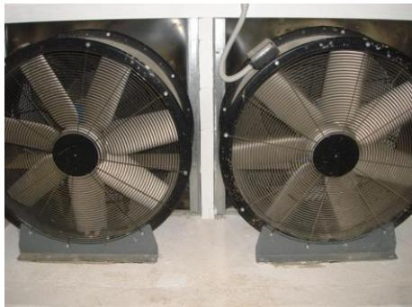
Ambient air is introduced through a buried duct system. When flowing through these channels, air temperature approaches the temperature of the surrounding ground. The temperature of the ground, according to studies, is stabilized to 9 meters deep at a temperature close to 20 ° C.
