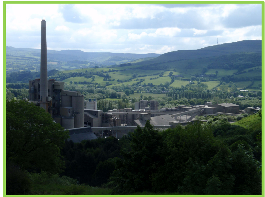
La Forge Cement Factory, Peak District (UK) Photo credit: Ruslan Zhechkov
