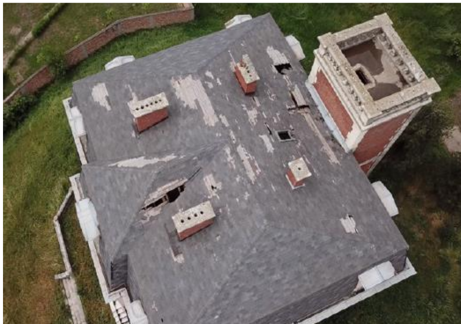
Before the intervention – June 2020
