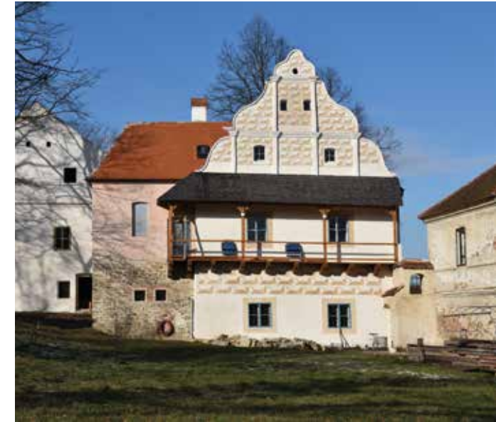
Mladějovice Mansion. Regional Development Agency of South Bohemia
