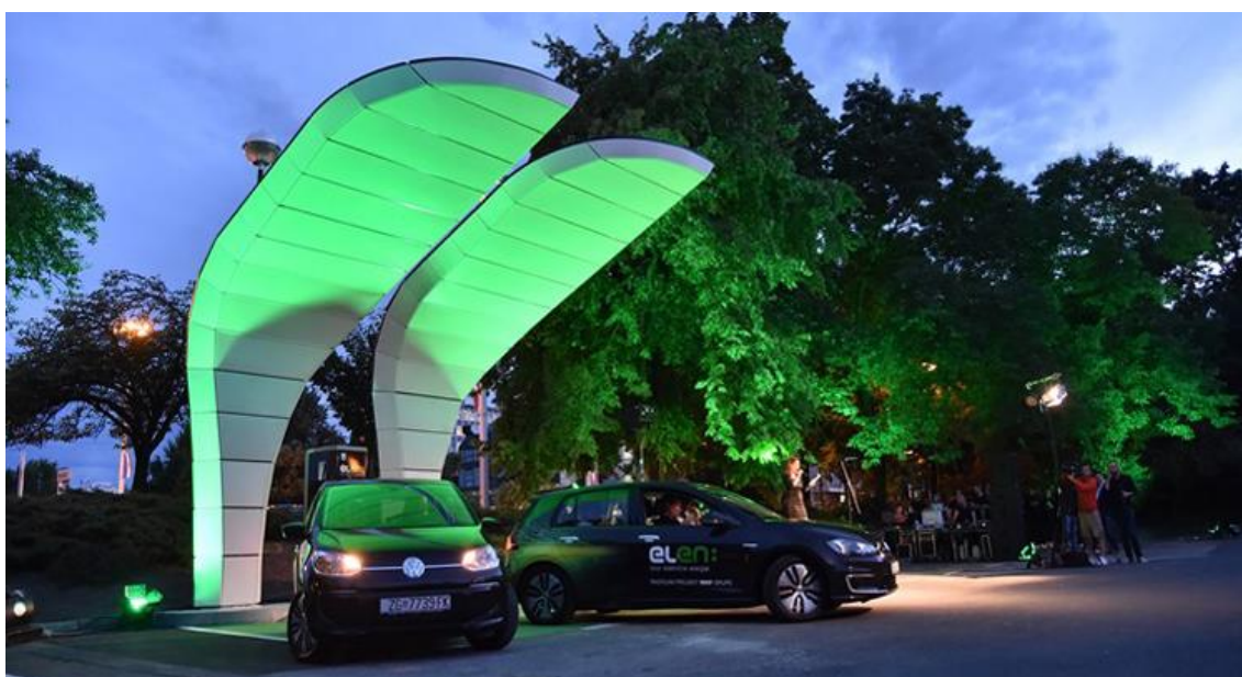
Figure 1 Canopy Charger with integrated photovoltaic power plant owned by HEP d.d. (Source: HEP d.d.)
