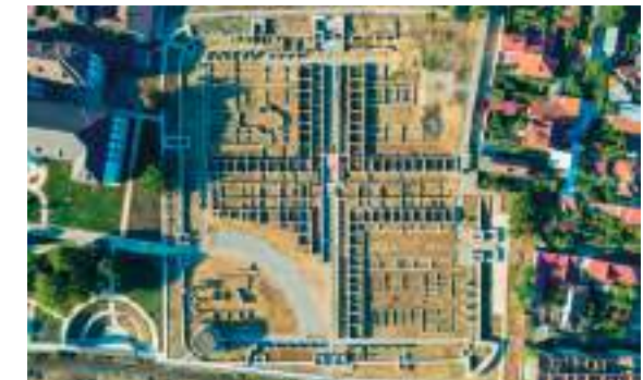
Iron Gates Museum aerial views. Dobreta Turnu Severin. Mehedinti County.
