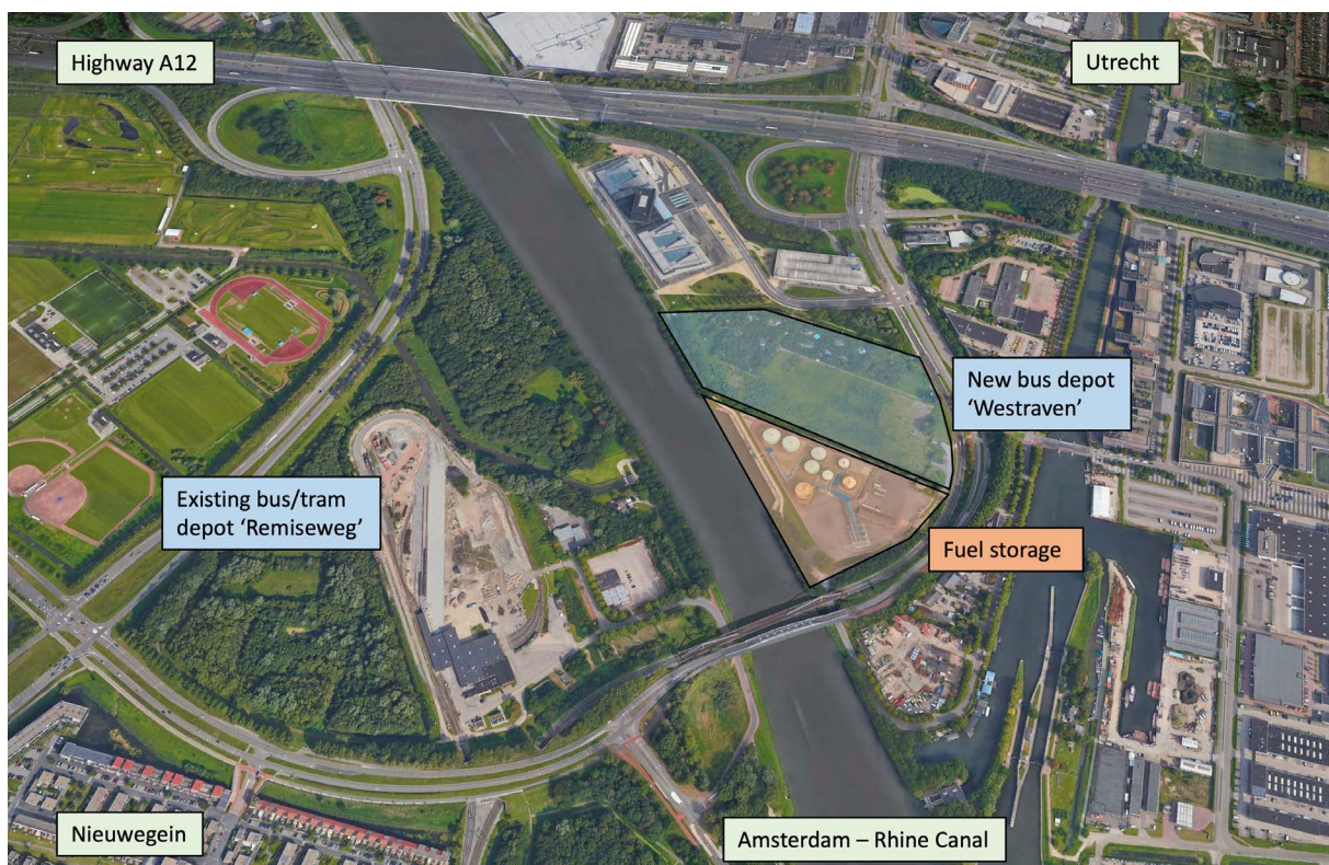
Situation bus depots and fuel storage at the Utrecht Westraven depot Source/data: Google Earth
