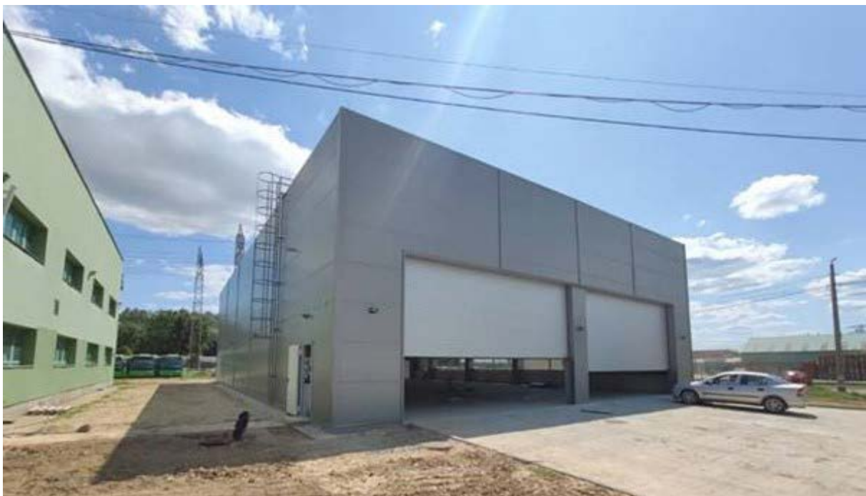
Hall building at Pécs (Source: B Build & Trade Ltd)
