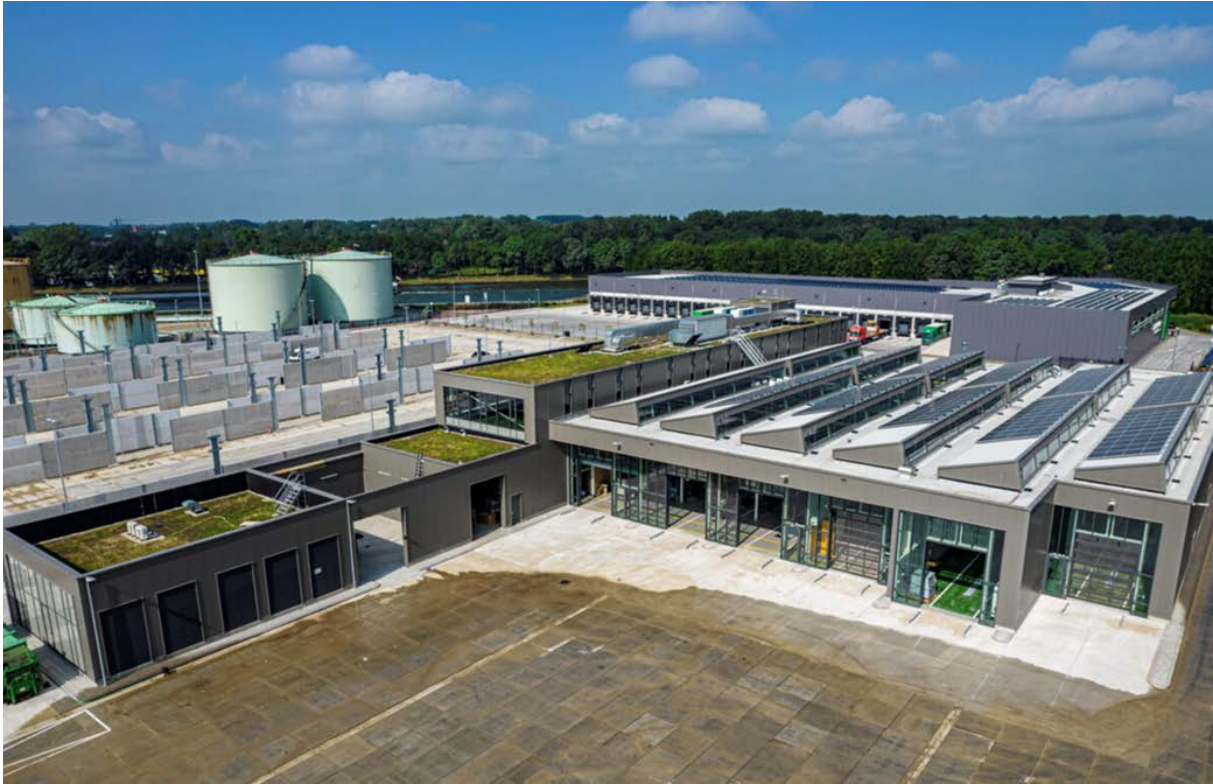
Bus depot 'Westraven' with the charging facility and the fuel depot on the left. Photo by Van der Ven, Brakel
