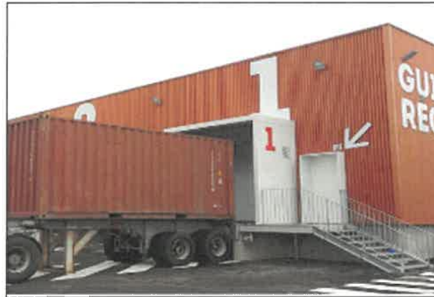
Figure 3, the "one stop shop" SIVEP facility in Montoir de Bretagne
