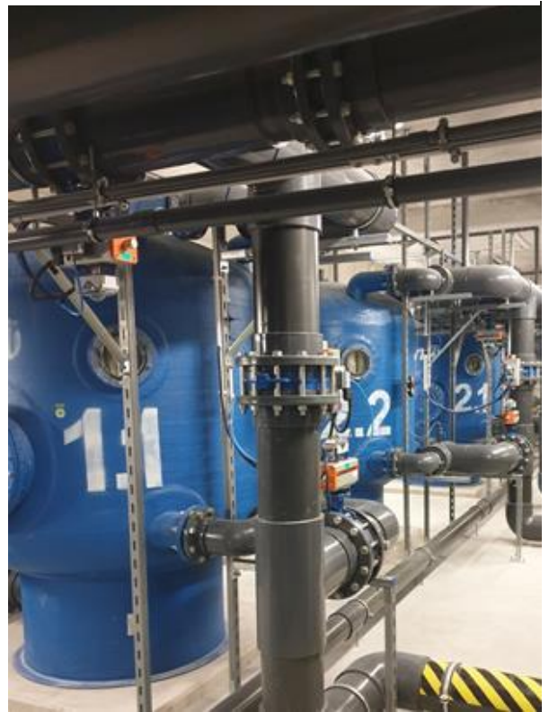
Figure 13 Pool basement tank which receives the water from the overflow gutters at the Łódź Sports Bay
