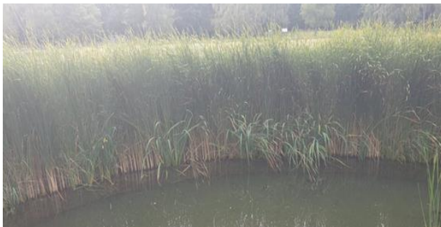
Figure 7 Rain water treatment layer for the inputs from low-usage land; it is filled with rocks and features water plants
