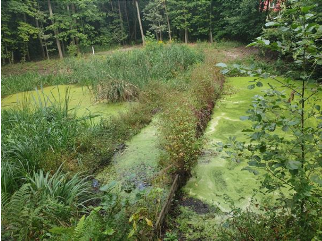
Figure 6 Sedimentation zone: treatment of water for sediment removal at a part of the system settling tanks
