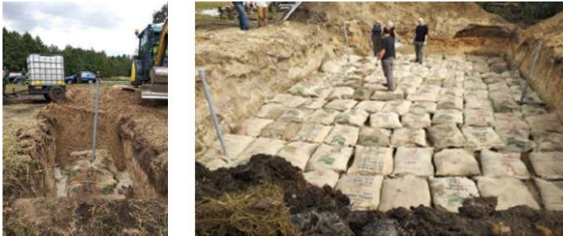
Figure 19 Horizontal modular OMP bed with the carbon substrate
