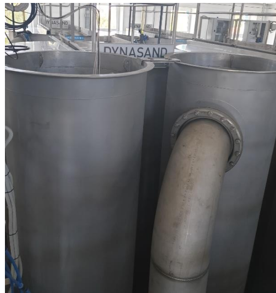
Figure 15 Water intake treatment at MPWiK Sieradz: DynaSand filters
