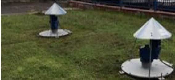
Figure 4 Membrane system installed at Janis
