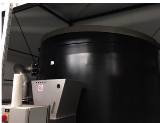
Figure 5 Averaging tank installed at Janis
