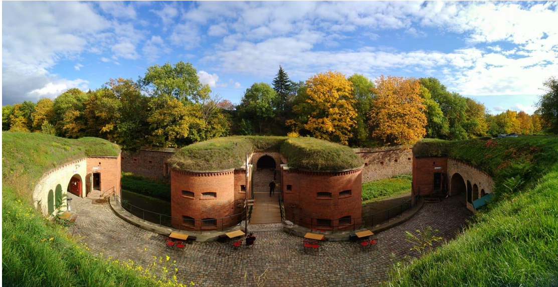
Figure 7: Ravelin II | Reconstructions through Volunteer Restoration Project "Sanierungsverein Ravelin 2 e.V."
