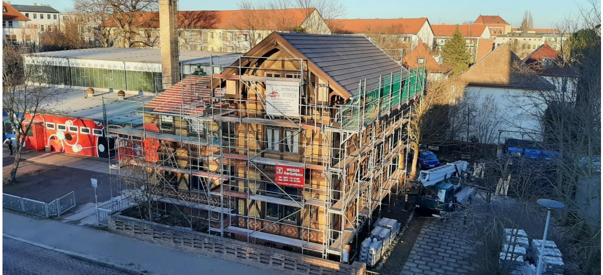
Figure 9: Rayon House currently under construction / Used as Pub and Beer Garden
